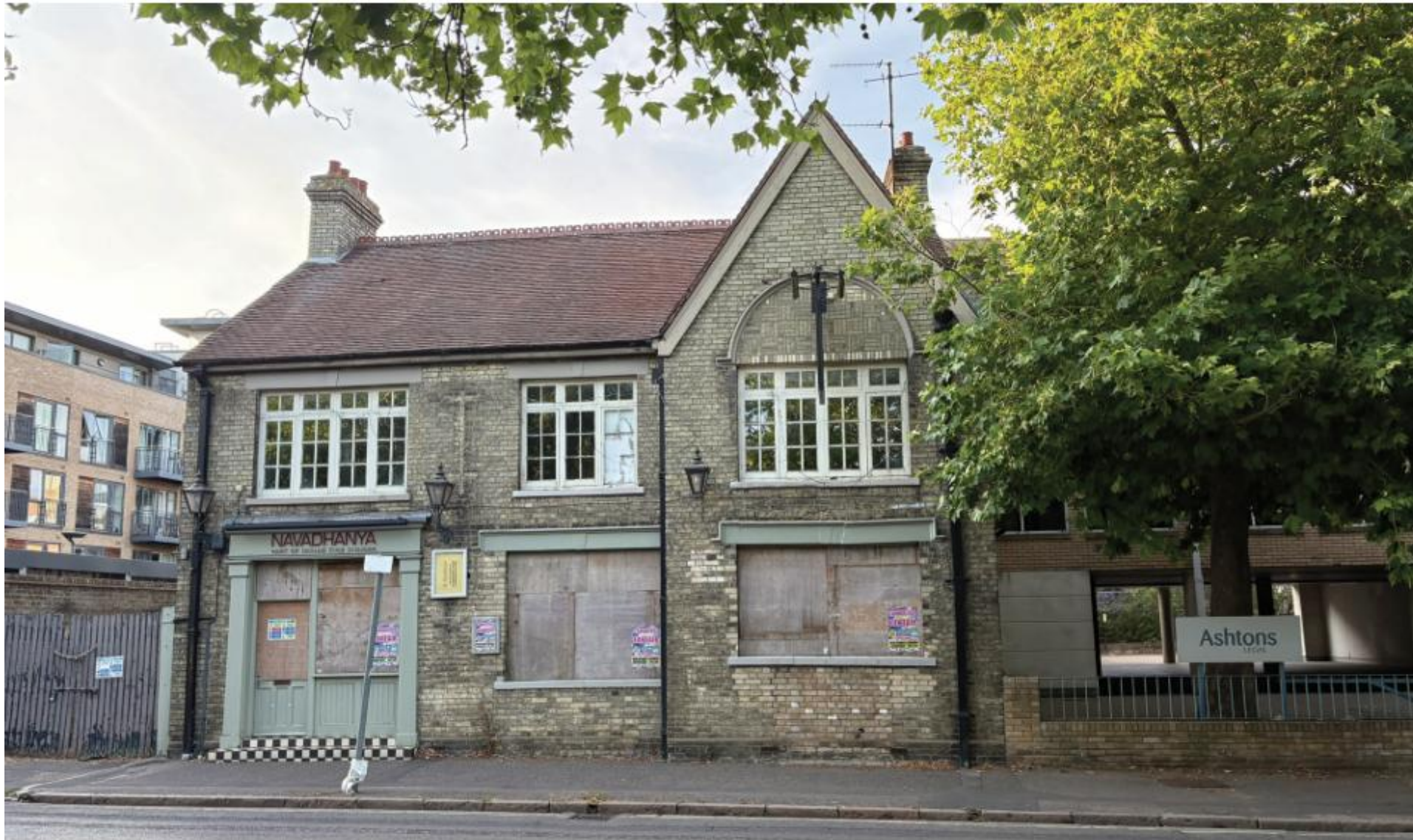
The existing building
